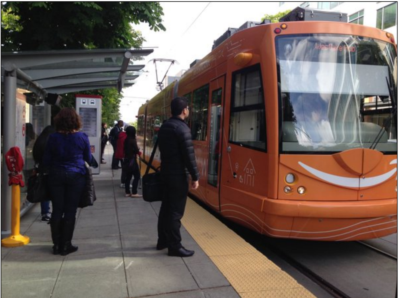
Figure 3: Streetcar station platforms provide a raised curb and level boarding areas for accessible boarding.
